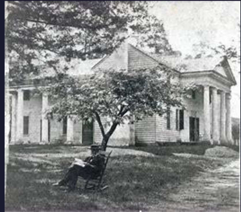
CLEMSON READING AT FORT HILL
